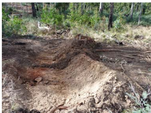
Photo - Grip on extraction track at coupe SFM134.
